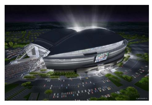
With spans typically ranging from 600 to well over a 1000 feet or more, these "long span" roof structures with moving roofs and playing fields present a host of challenges ranging from the economics of spanning long distances with moving loads, the constructability aspects of putting the steel structure in place and the wind loading that such buildings receive depending on their roof configuration - open or closed. How are these enormous
