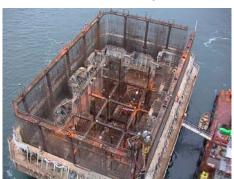
The original bridge, made famous as "Galloping Gertie", was, at the time it opened in 1940, the third longest suspension bridge in the world. The superstructure of the first bridge collapsed in a relatively minor windstorm within 4 months of its opening. It was rebuilt in 1950. The foundation of the new bridge, like the old, consisted of two deep concrete caissons which were constructed while floating and then sunk into the sea bottom using open dredge well techniques.
