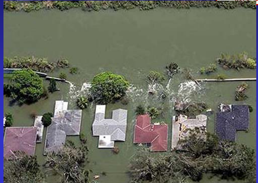
London Ave. Canal Breach at Robert E. Lee Blvd.
