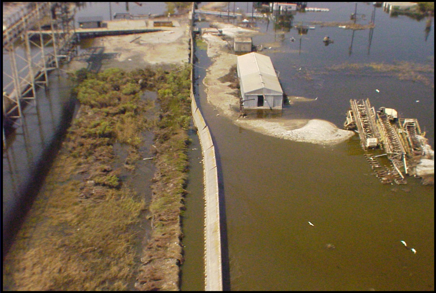
Citrus Back Levee – NOE04
