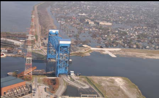
Northern 9 th Ward Breach
