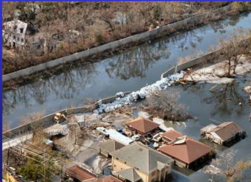
London Ave. Canal Breach at Mirabeau Ave.
