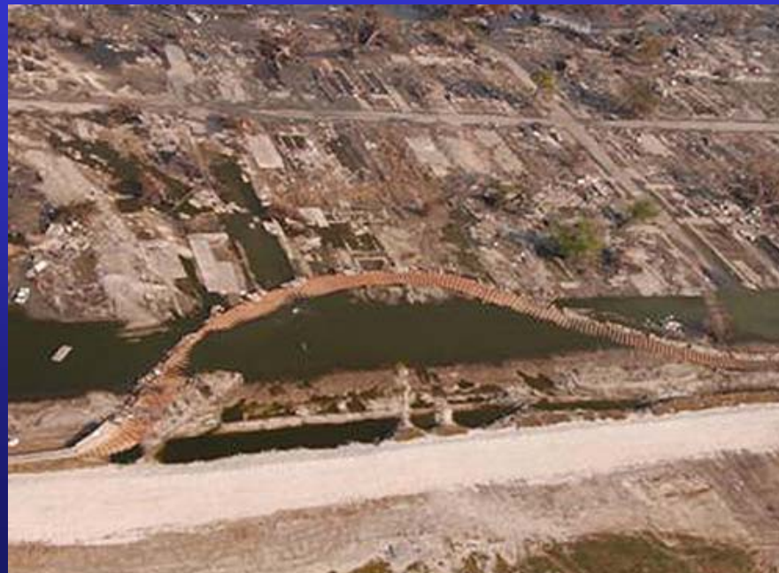
Sheetpile Floodwall Collapse – 9 th Ward (East Side)
