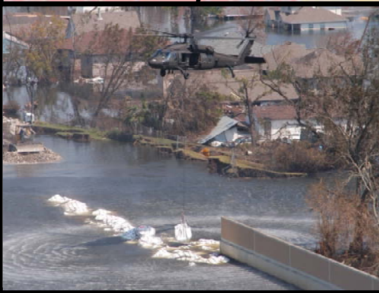
17th St. Canal I-wall Breach
